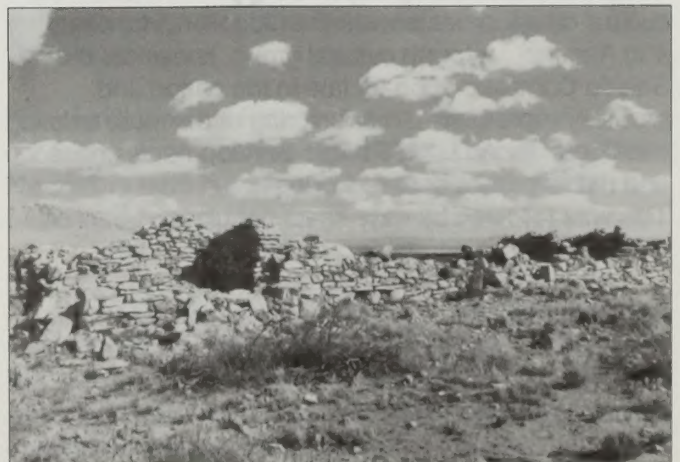
Ruins of a Butterfield Stagecoach station are located near the Peloncillo Mountains.
